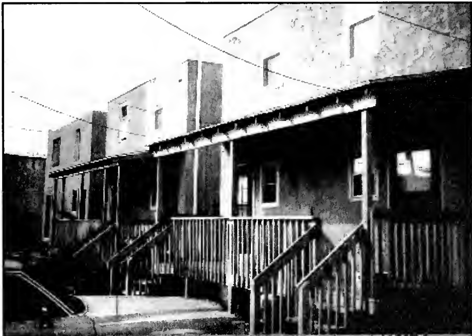
Figure 9: Rear view of houses after Clinton Street rehabilitation. Photo courtesy of Metro Camden Habitat for Humanity.
